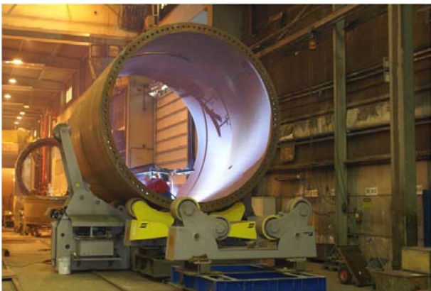
Figure 4. The tower section is assembled from a number of tower shells. The photograph shows a fitting and tack welding station (source: Levator Oy).
