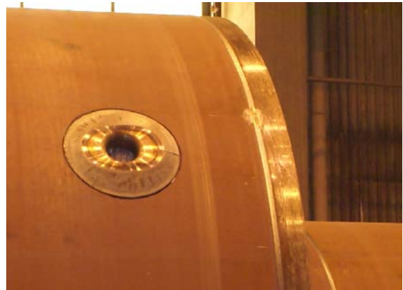
Figure 5. The flange of the aircraft warning light fitted in place (source: Levator Oy).
